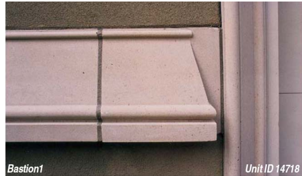
Here is an example of a backed cope. This allows a smooth end of a profile
