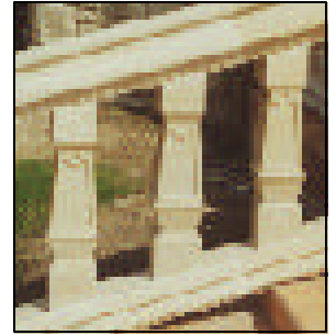
EXAMPLE PHOTO OF BALUSTRADE STAIR
