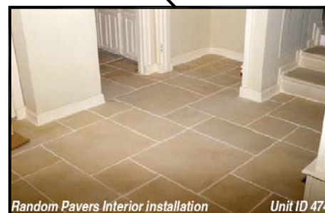
Random Pavers interior installation
