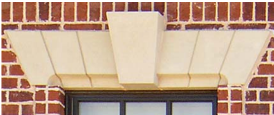
The angles give a unique design to this Jackarch with a Flatfaceslant Keystone.
