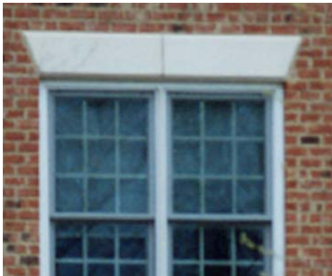
An example of an extruded Jackarch over a window
