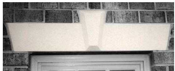
This example shows the Jackarch with a very popular chamfer keystone.
