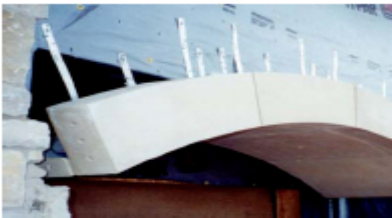
Suspending the stone with straps.
