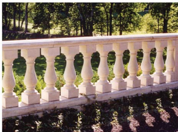
At left is a photo of Otterwood1 Extrados1 Chamfer1 Balustrade set on 12" centers. Compare with the illustration of standard installation above.
