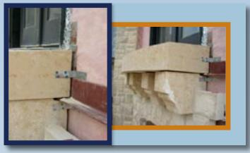
L-Clips & Tapcon screws secure the stone in position. Steel beams support and distribute the weight
