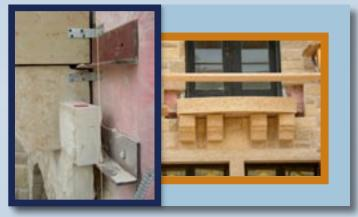
A plumb line stages the offset of the surrounding veneer as it finishes out the window sill.
