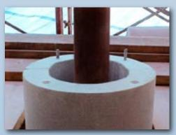
Precast holes are set with pins to alight the column sections
