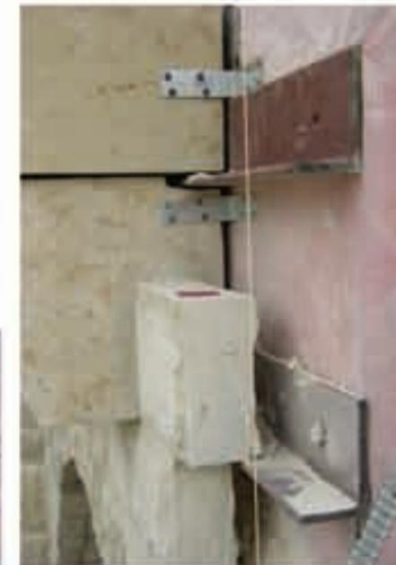
Left and above, an excellent example of clip anchors and steel lintels used in a surround installation.
