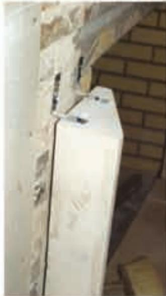
Left, a fireplace leg using strap anchors and tapcon screws.
