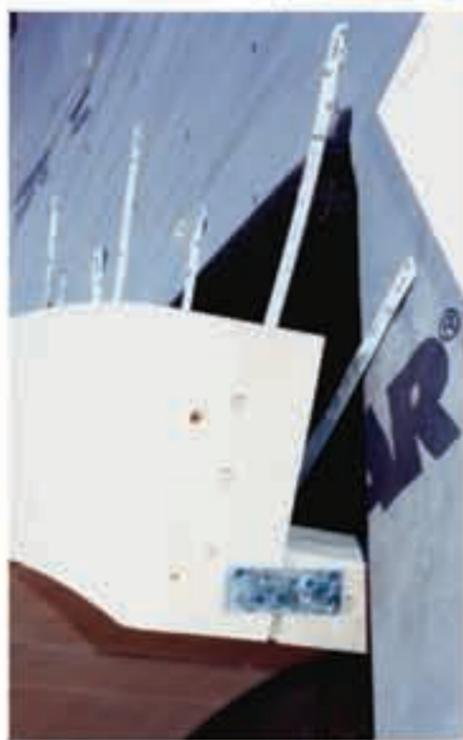
Left and above, securing a circletop surround with soffit using strap anchors and tapcon screws.
