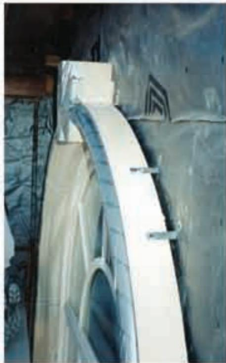
Above, securing a circletop surround using strap anchors and tapcon screws.
