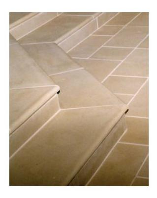
**Steps** - The step is composed of the tread and riser. Tread - The part of the stairway that is stepped on. Riser - The vertical portion between each tread on the stair.
