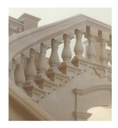
**Balustrade** - An entire railing system as along the edge of a balcony or stair. Includes top rail, balusters, and a bottom rail. Runs of balustrade are occasionally seperated by newel piers.
