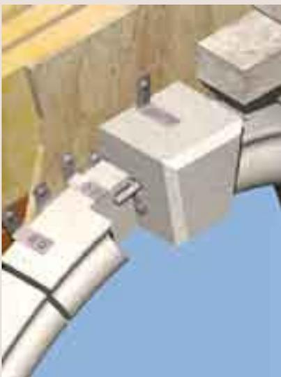
Pins align the units and L- clips attach to the edge of the stone.
