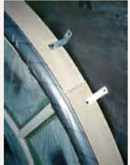
Note the protective tape covering the stone face to prevent any mortar spillage from staining the stone pieces.
