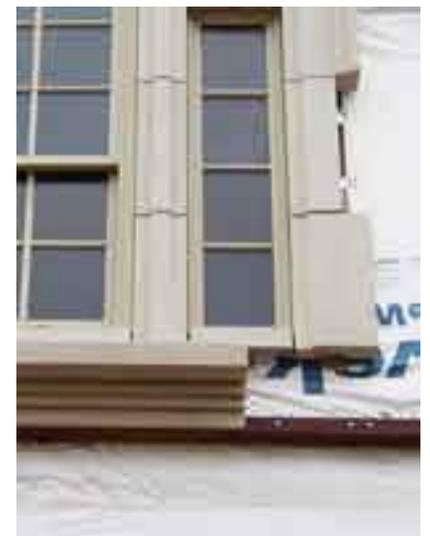
Steel beams offer support for the sill as it is prepared for mortaring.
