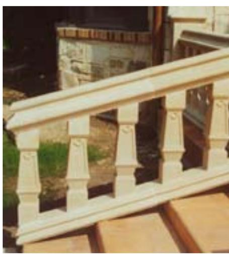
(baluster) (handrail) (baserail)
