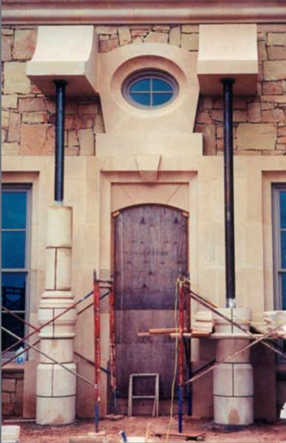
Custom hollow columns installed with steel pipe reinforcement.
